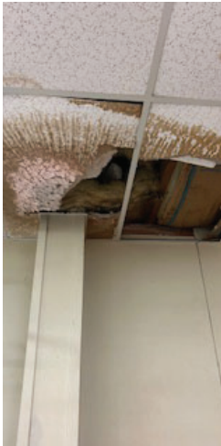
Damage from Leaking Roofs
